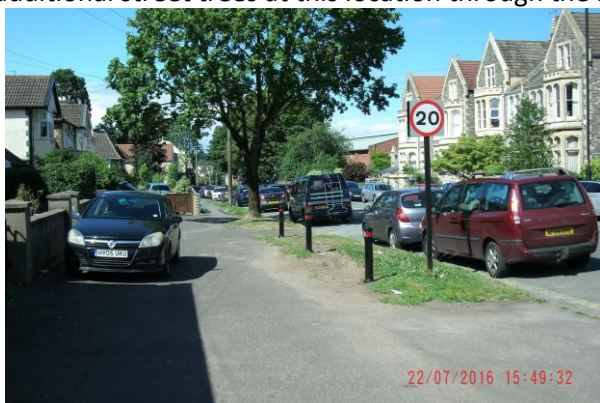
Westbury Road Bollard Installation
